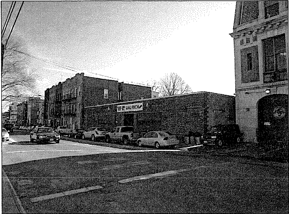
View to the project site from 43rd Avenue 2
