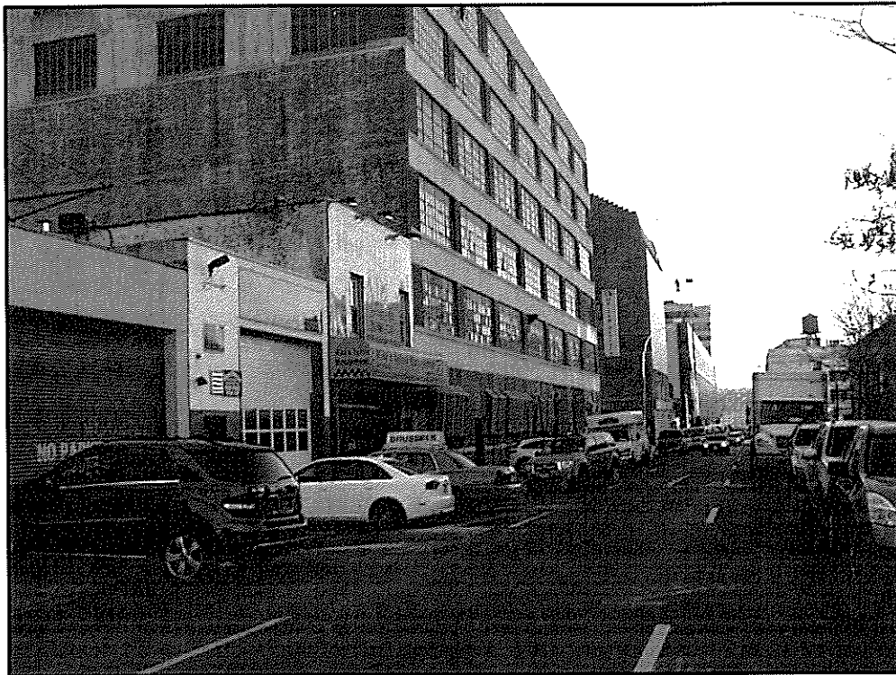
Photo 2 – Looking west toward Eleventh Avenue on West 44th Street
