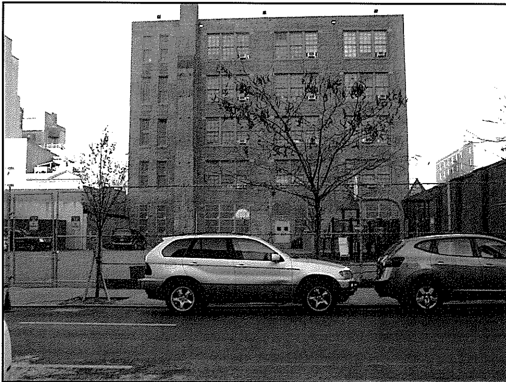
Photo 4 – Rear View of PS 51 from West 44th Street
