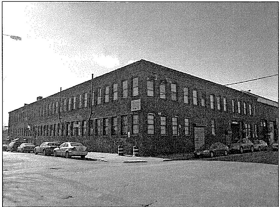
Former Tiffany Studios Complex - Southwest corner of 43rd Avenue and 97th Place
