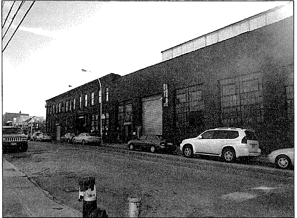
View east on 43rd Avenue to a warehouse building complex 8
