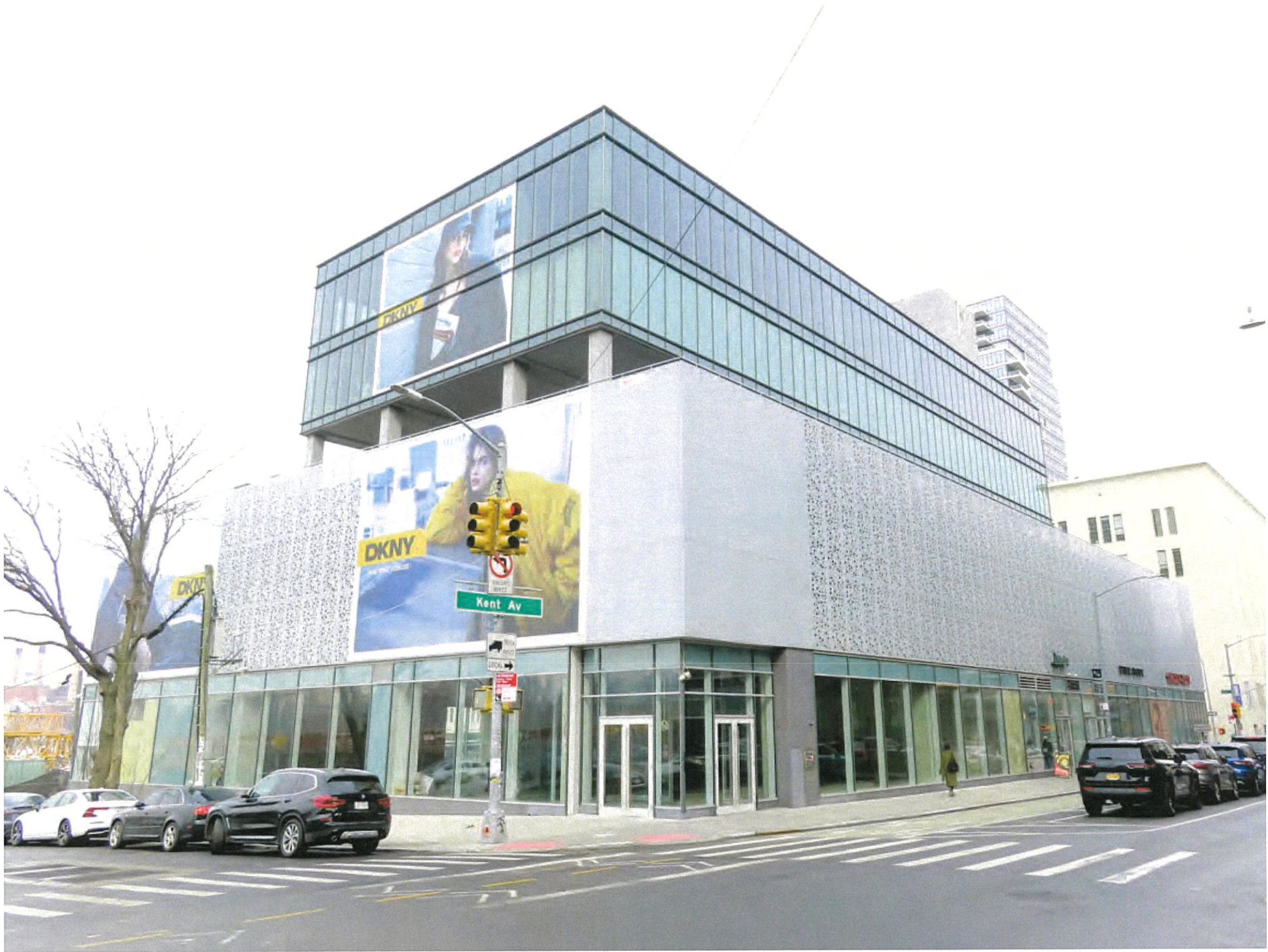
View of the Development Site facing North from the intersection of Kent Avenue and Metropolitan Avenue
