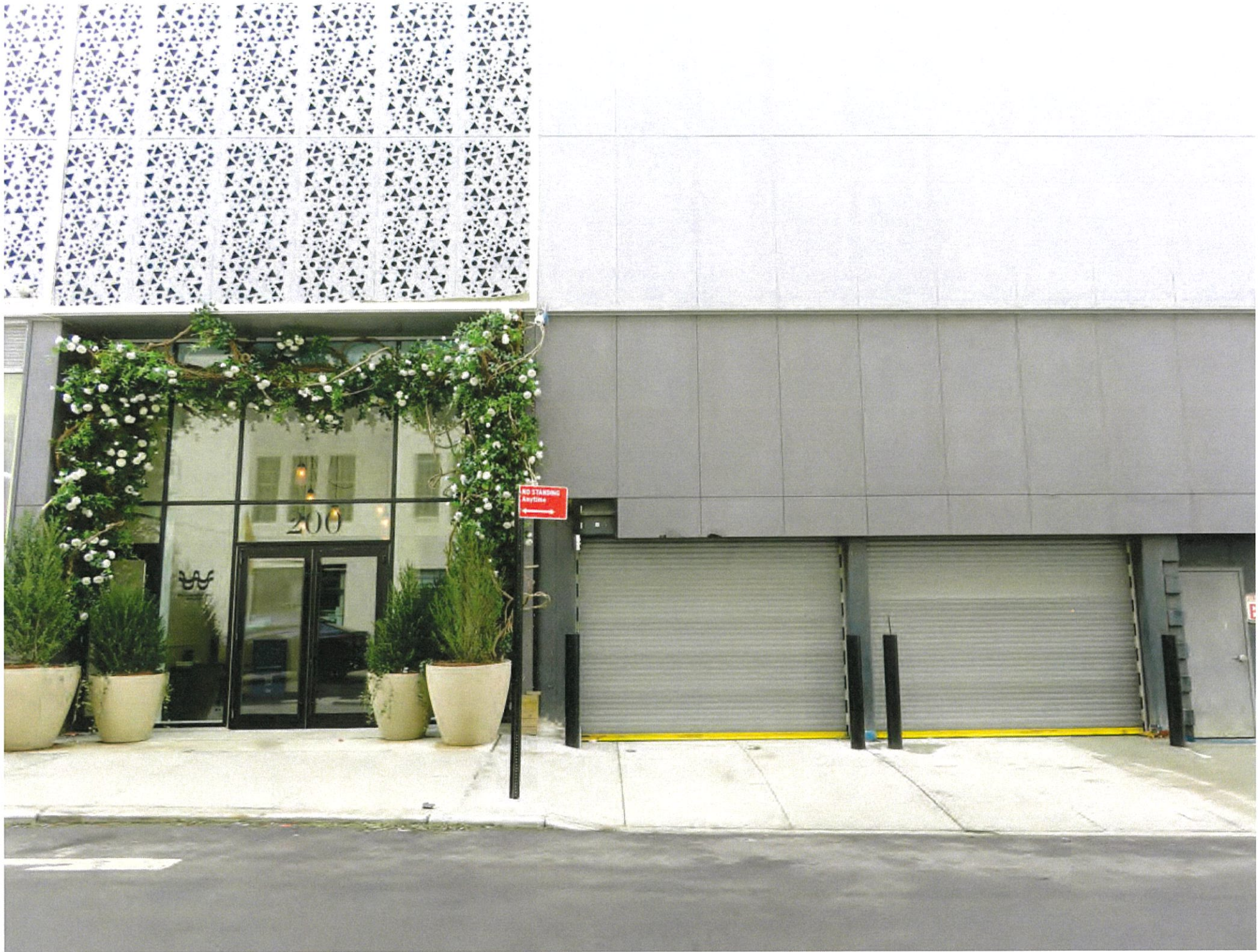
View of the Development Site facing Southwest from North 3rd Street
