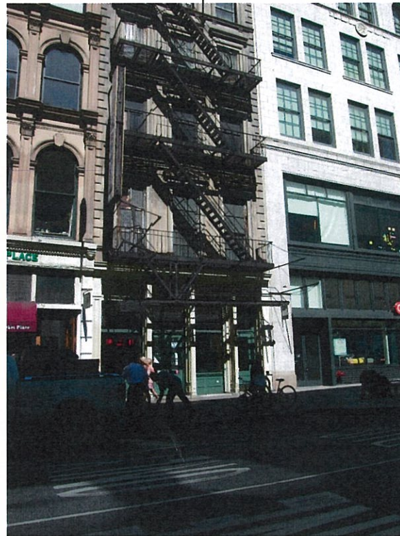
03 VIEW SOUTHEAST OF BROADWAY TOWARDS BUILDING FACADE
