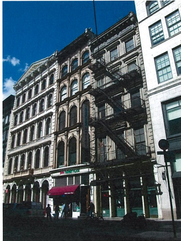
01 VIEW NORTHEAST OF BROADWAY TOWARDS BUILDING FACADE
