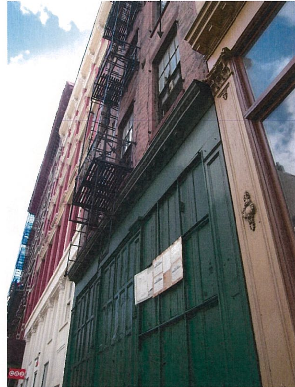
06 VIEW SOUTHWEST OF BROADWAY TOWARDS BUILDING FACADE
