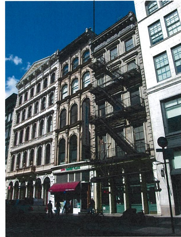
04 VIEW NORTHEAST OF BROADWAY TOWARDS BUILDING FACADE
