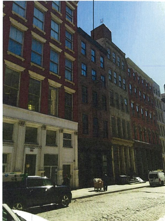
05 VIEW NORTHWEST OF MERCER ST. TOWARDS BUILDING FACADE
