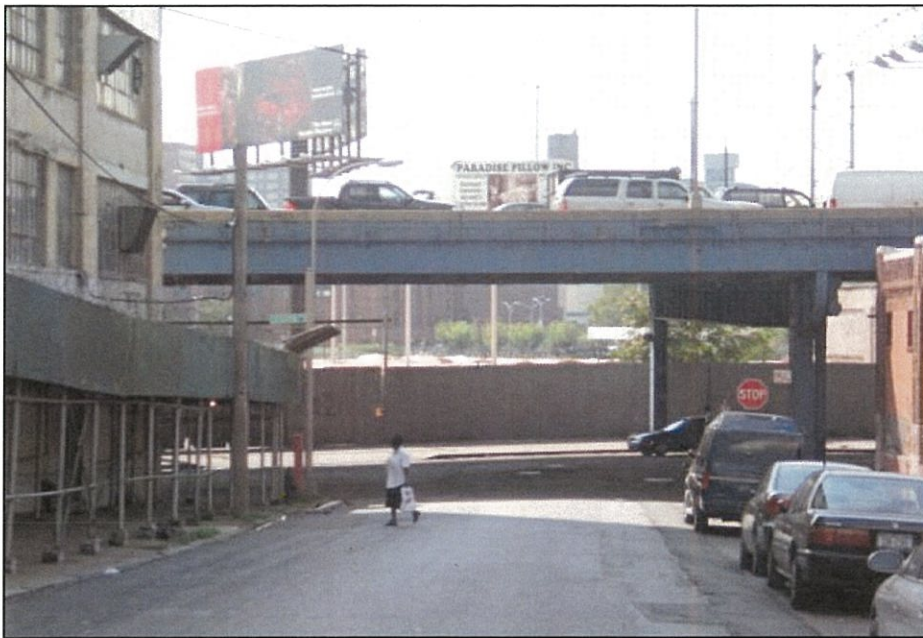
Elevated Major Deegan Expressway
