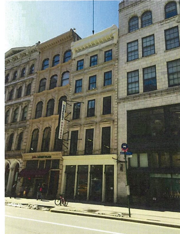
04 VIEW NORTHEAST OF BROADWAY TOWARDS BUILDING FACADE
