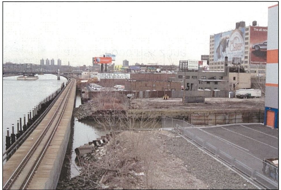
Oak Point Rail Link waterside
