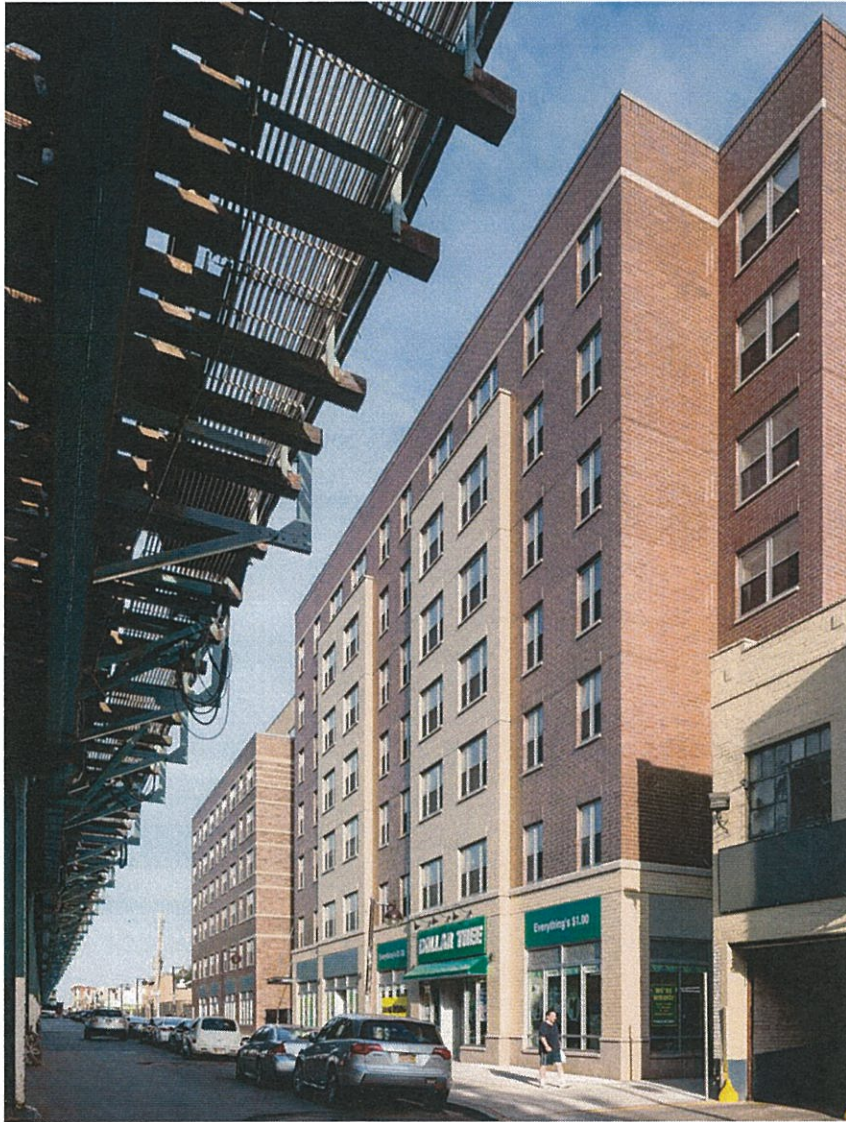
Eastward looking towards Olmstead Ave.
