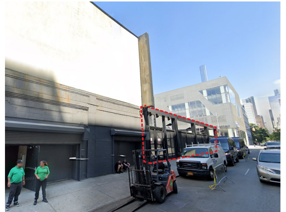
4. VIEW FROM W 55TH ST SW
