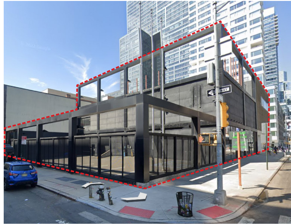
1. VIEW FROM 11TH AVE S
