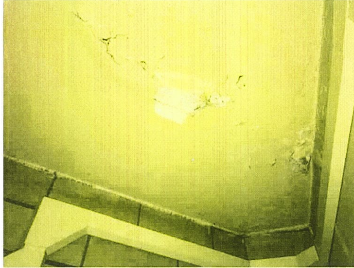
Photo 9: Close up view of a typical slab underside at 17 th floor hallways where the hammer tests revealed several areas of unsound concrete.
