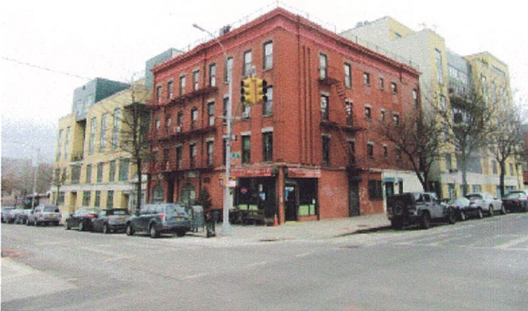
6. View of the intersection of Underhill Avenue and Dean Street facing northeast.
