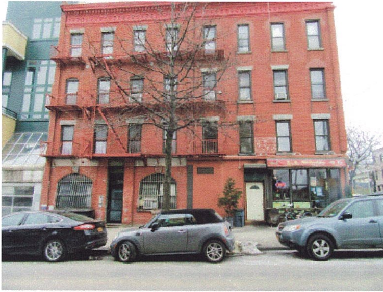
4. View of the side of Underhill Avenue facing east between Pacific Street and Dean Street.
