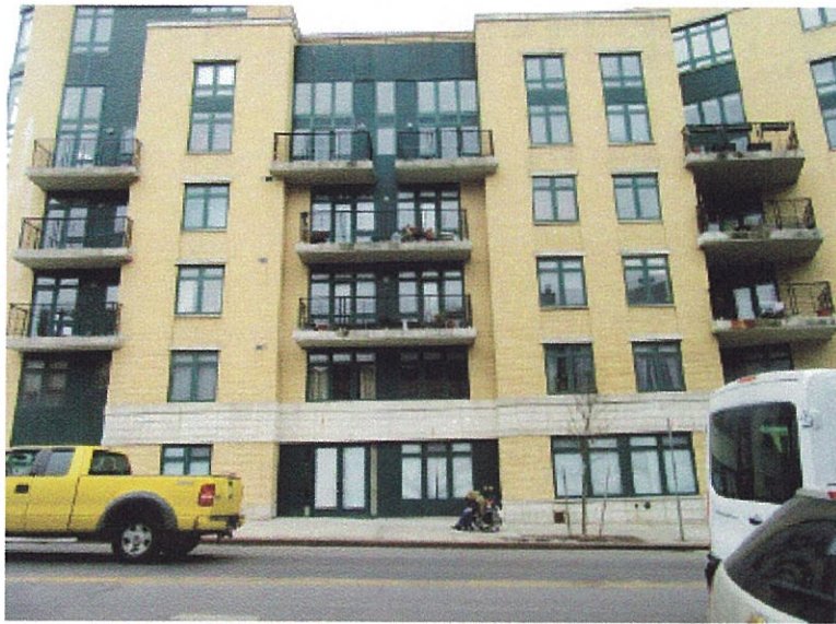
16. View of the Site facing west from Washington Avenue.
