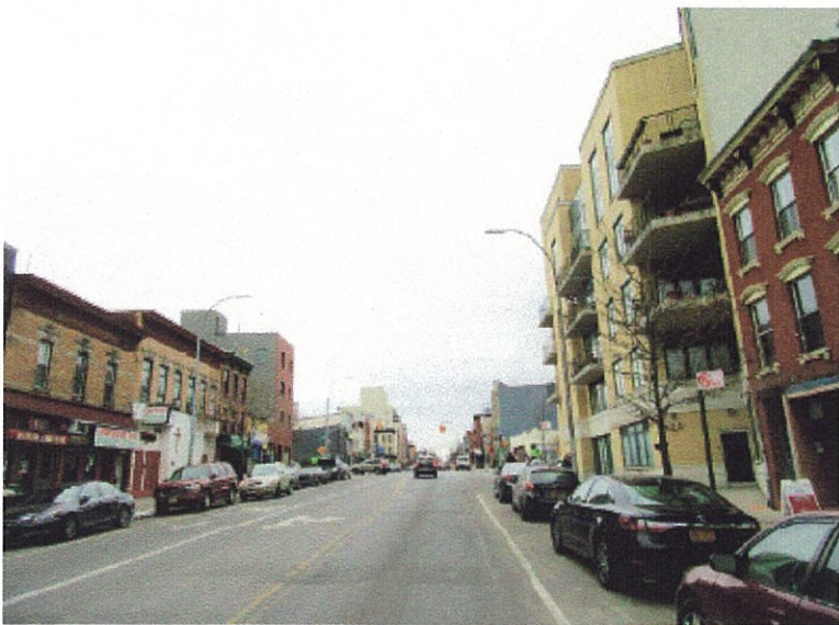
18. View of Washington Avenue facing southeast (Site at right).
