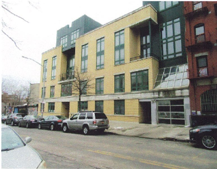
1. View of the Site facing northeast from Underhill Avenue.
