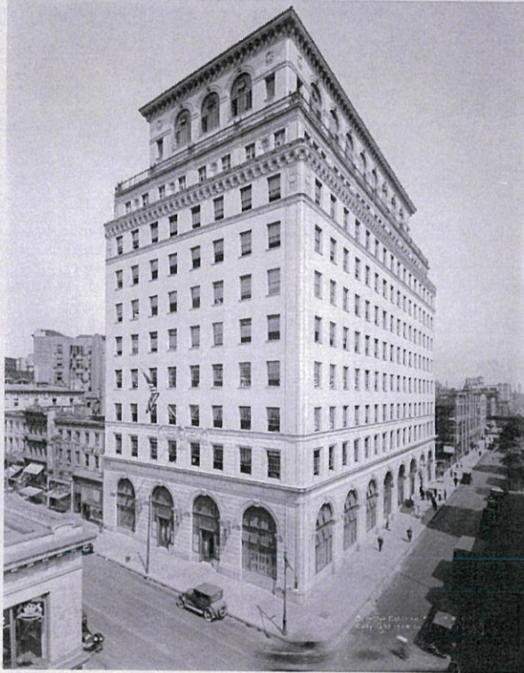
The Brooklyn Edison Building West Facade, 1924, Brooklyn Museum
