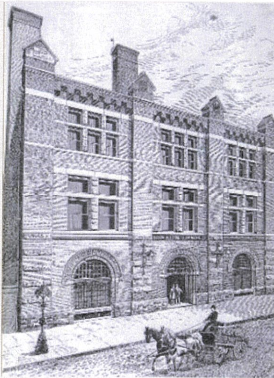
The first station of Edison Electric Illuminating Company of Brooklyn at 360 Pearl Street, Thomas Edison National Historical Park, via IEE Power and Energy
