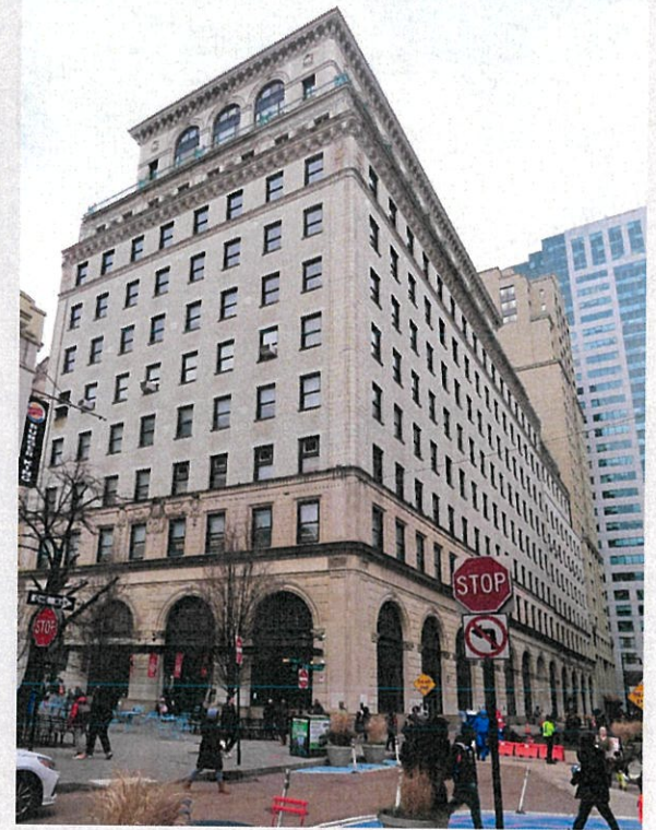
Brooklyn Edison Building, 2024, LPC
