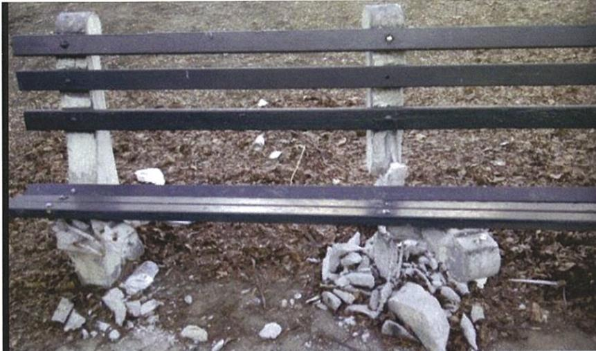
*Repairing bench slats does not stop from the old concrete crumbling.
