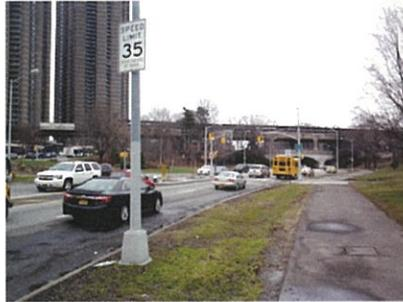
It should be possible to remove at least one lane in each direction. Narrowing the roadway will encourage traffic to slow, and will provide additional space for landscaping
