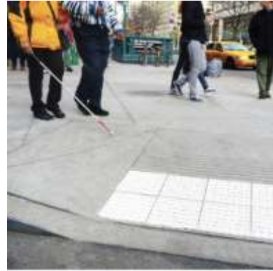
ADA accessible crosswalk in Columbus Circle, Manhattan
