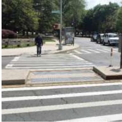
ADA accessible crosswalk on Claremont Parkway & Crotona Avenue, Bronx
